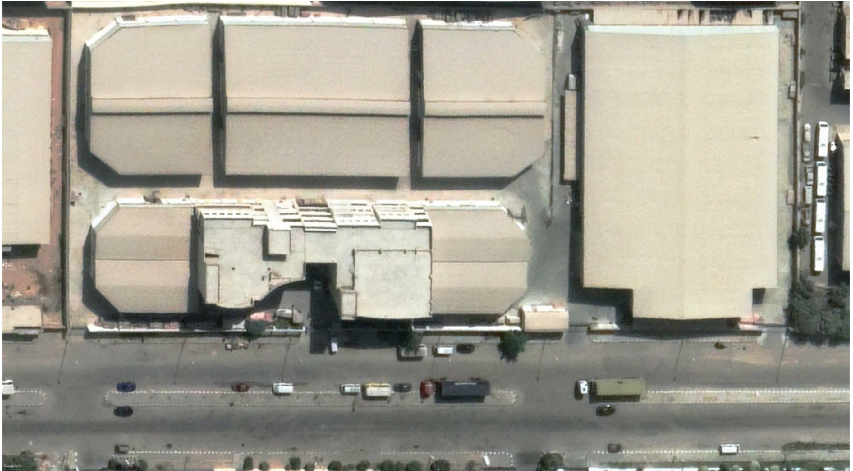
Production facilities in Badr City-Cairo
